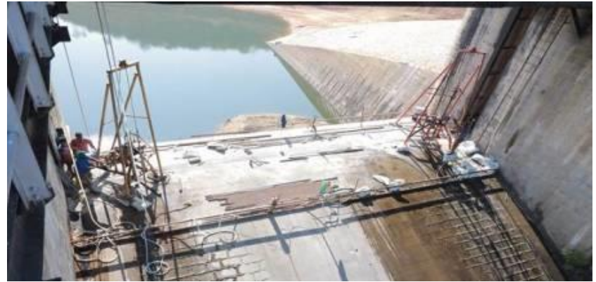
Core Drilling activity in spillway portion of Sholayar Dam
