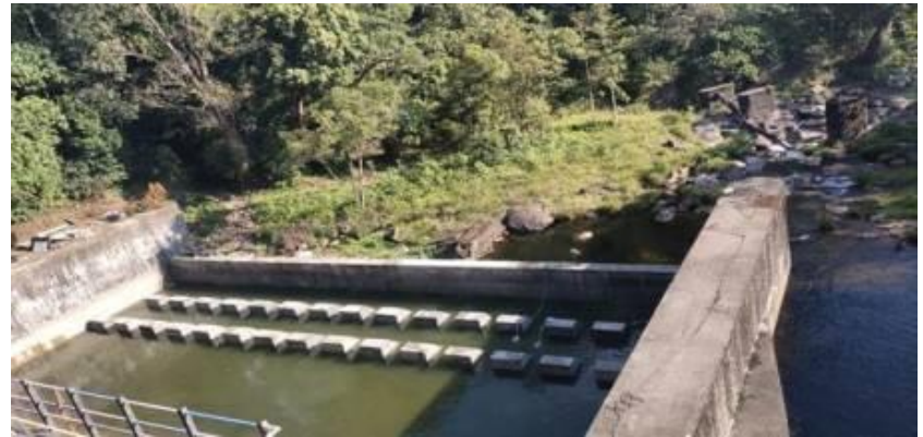
Stilling Basin at Upper Nirar weir
