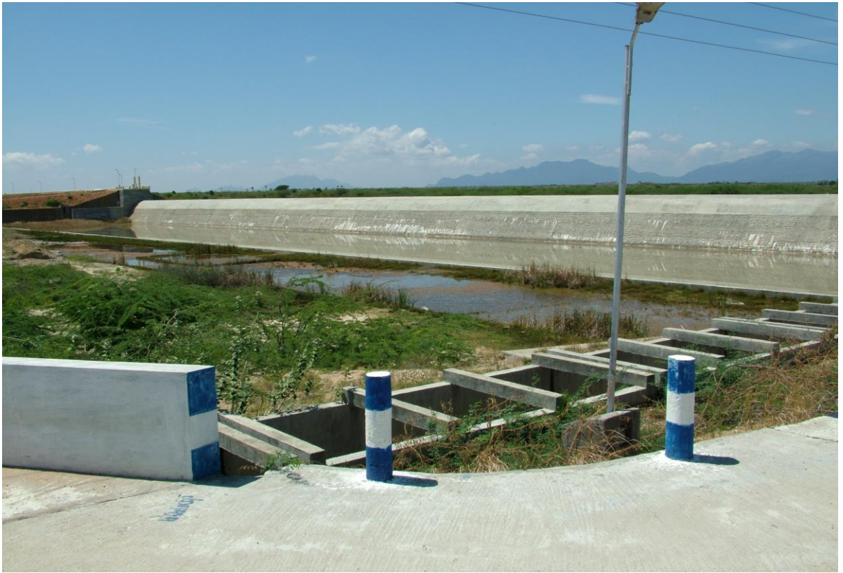
D/S view of Nambiyar Reservoir
