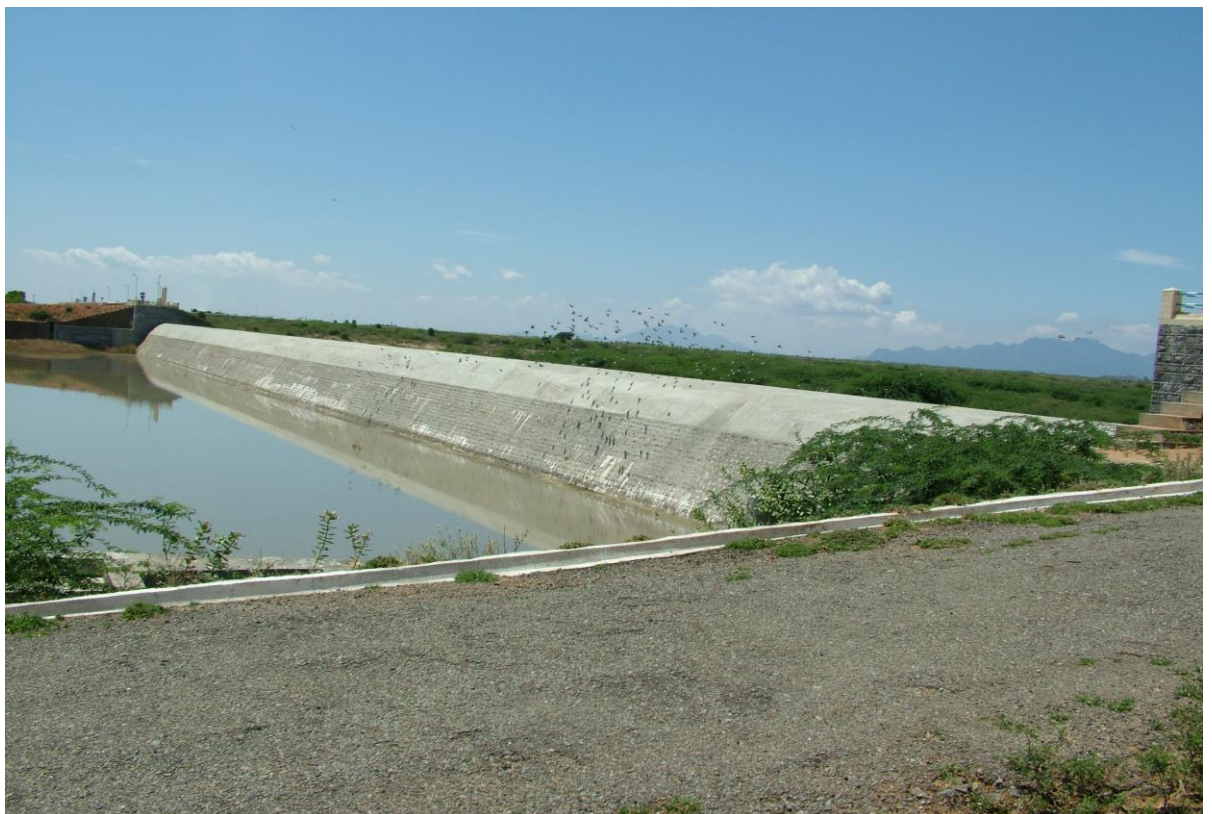
D/S view of Nambiyar Reservoir
