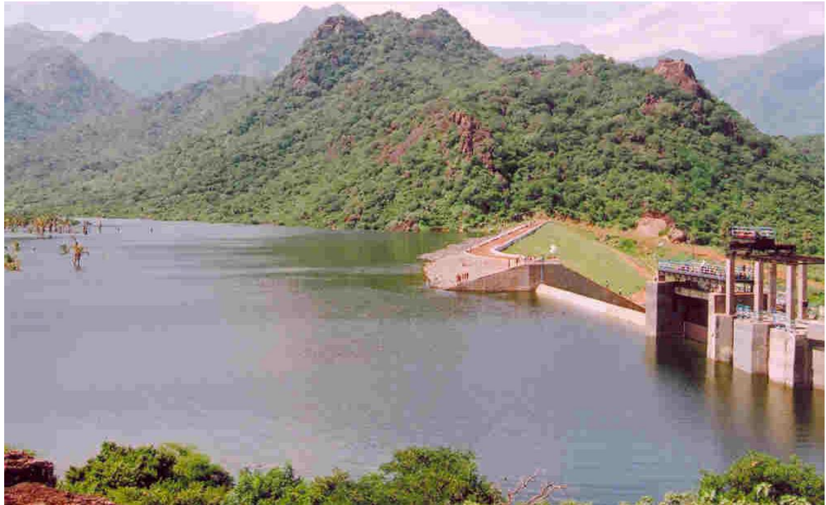
U/S View of Kodumudiyar Reservoir
