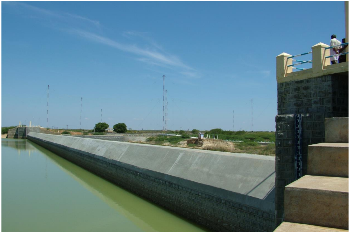
U/S view of Nambiyar Reservoir
