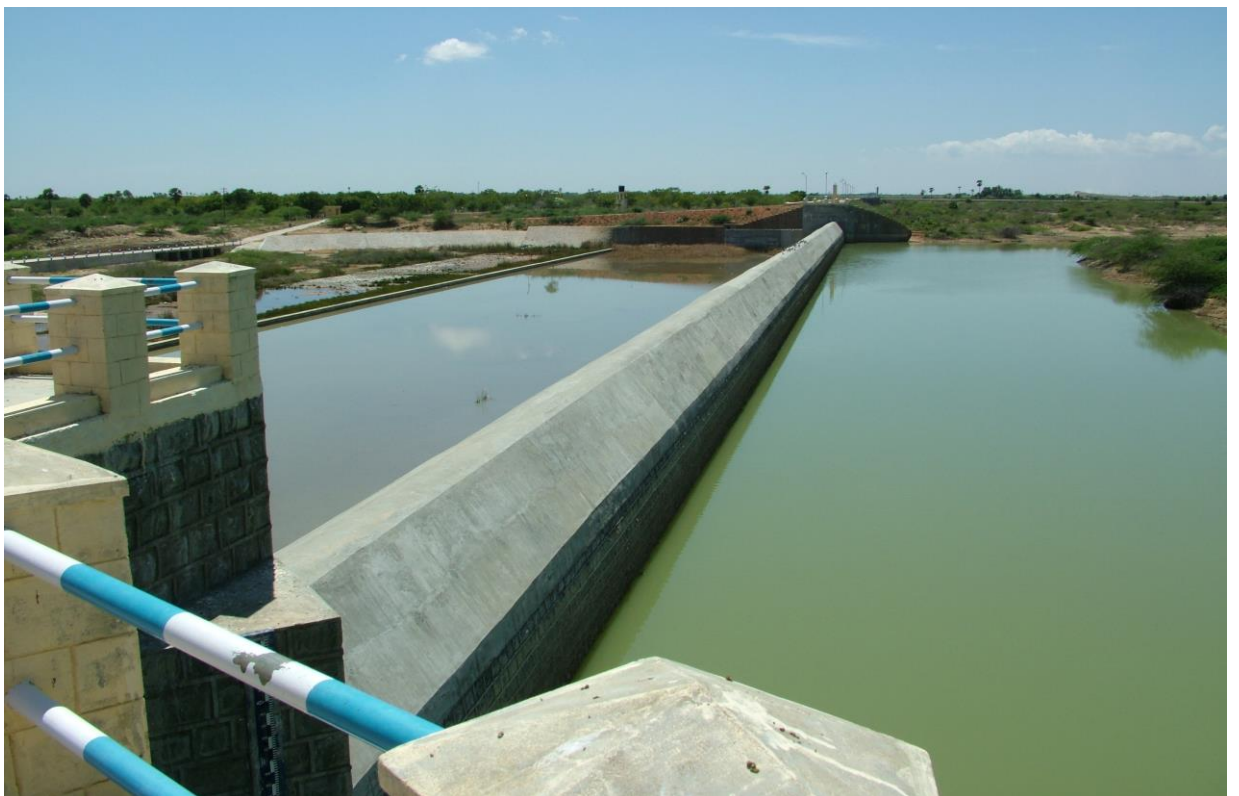
U/S and D/S view of Nambiyar Reservoir
