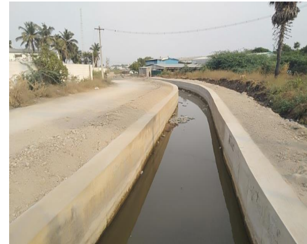
Retaining wall in Andipalayam Supply Channel
