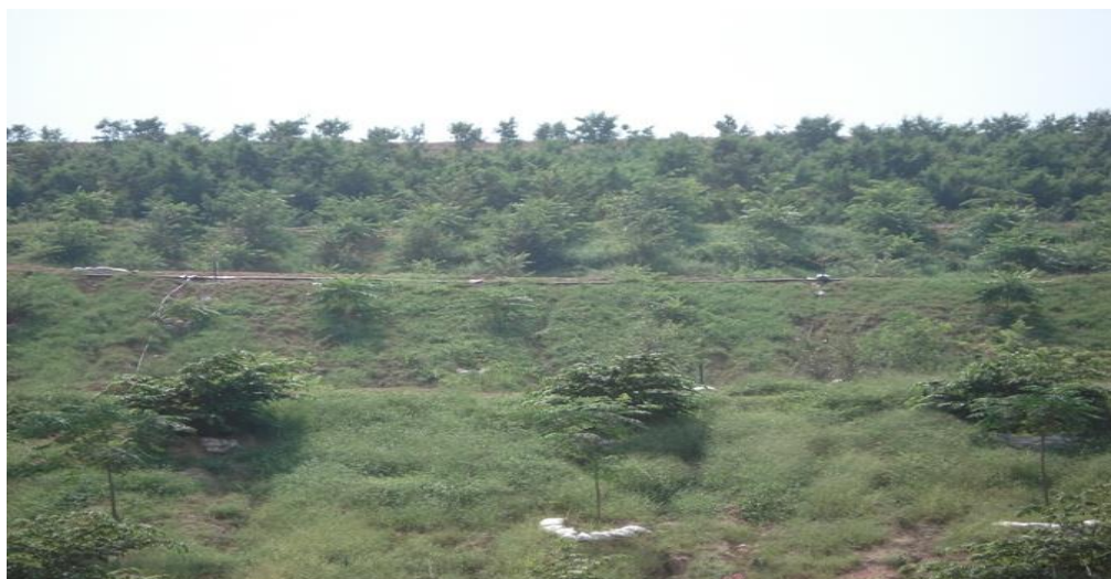
Fig 9.9 Slope Stabilization by Afforestation
