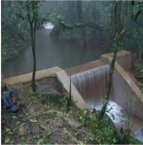
Fig 9.4 SILT DETENTION STRUCTURE
