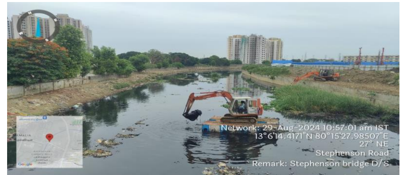
DURING EXECUTION Stephenson Bridge D/s
