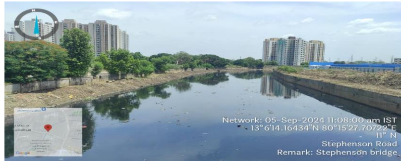
DURING EXECUTION Stephenson Bridge D/s
